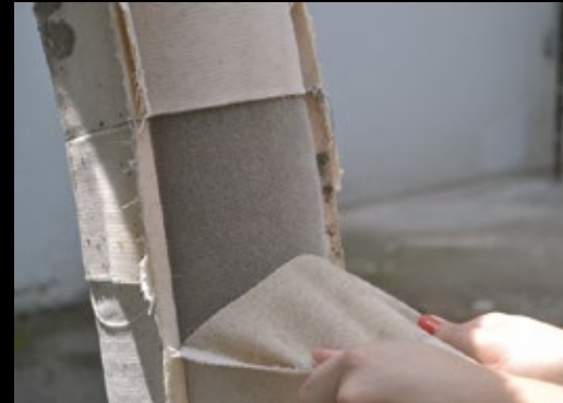
ARTESANA L CONCEPT- INSPIRATION WORK BY DANIEL A SOLIS Textile formwork technique.
